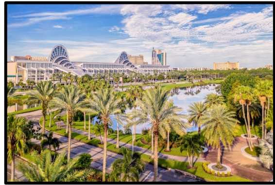
The OCCC North-South Building.
